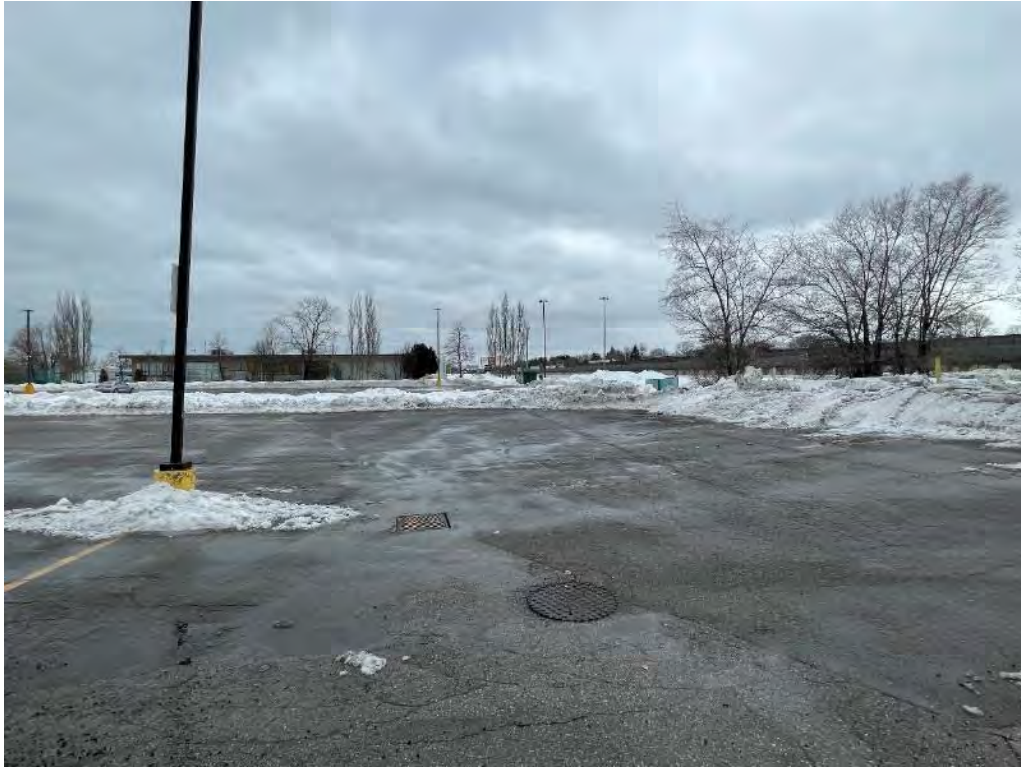
Photo 13: Parking lot in the northwestern portion of the Site, facing west.
