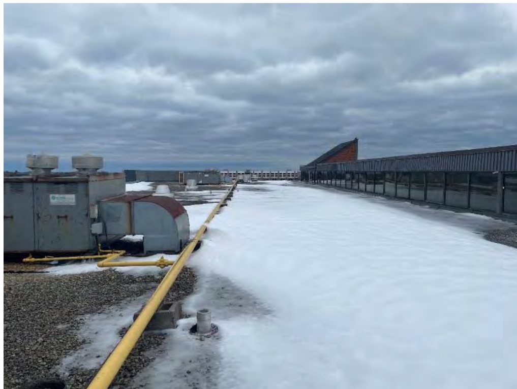
Photo 4: Roof of Site building, facing east.
