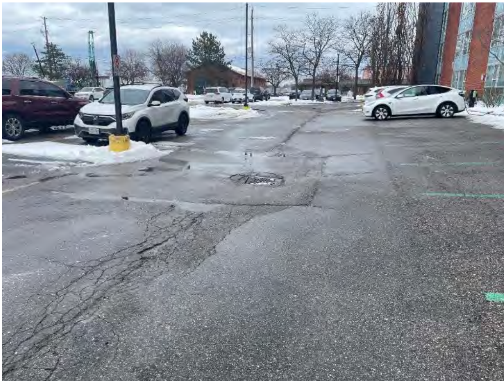
Photo 12: Parking lot to the east of the Site building, facing south.
